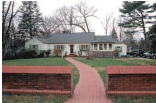
950 Belvidere Avenue Plainfield $539,000
