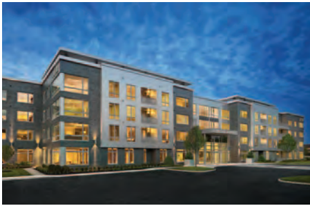
90 Park Avenue Florham Park
